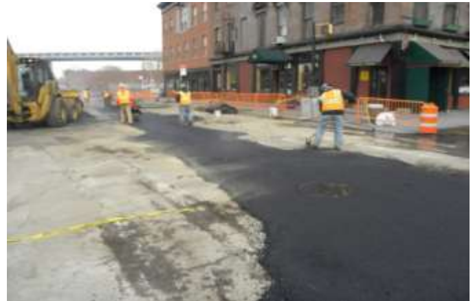
Temporary paving of roadway on Water Street at Old Fulton Street.
